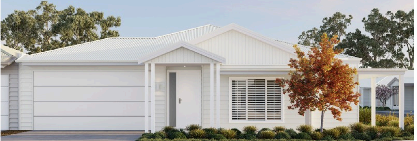
Corner Facade scheme: Coastal White
